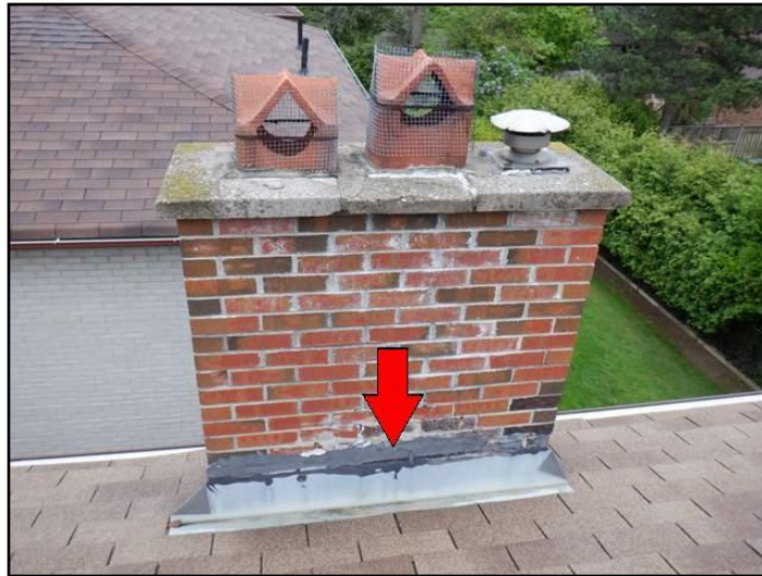
Prior repairs. Sealant deteriorated
