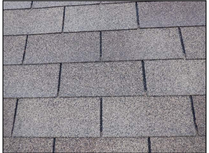
Asphalt shingles
