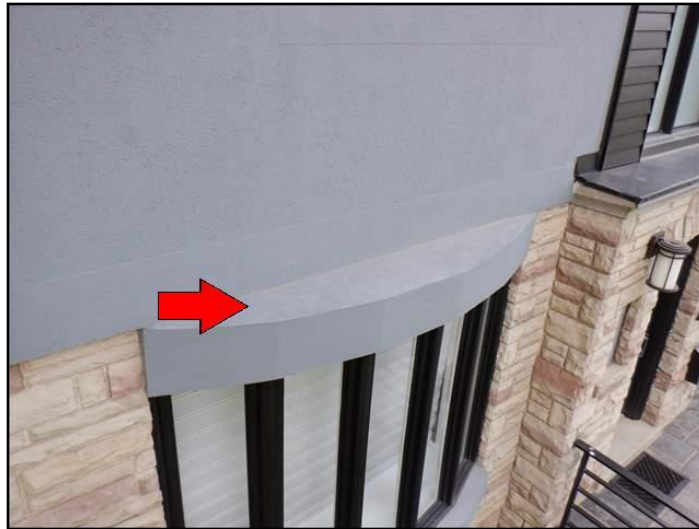
Exterior Insulation Finishing System (EIFS)
