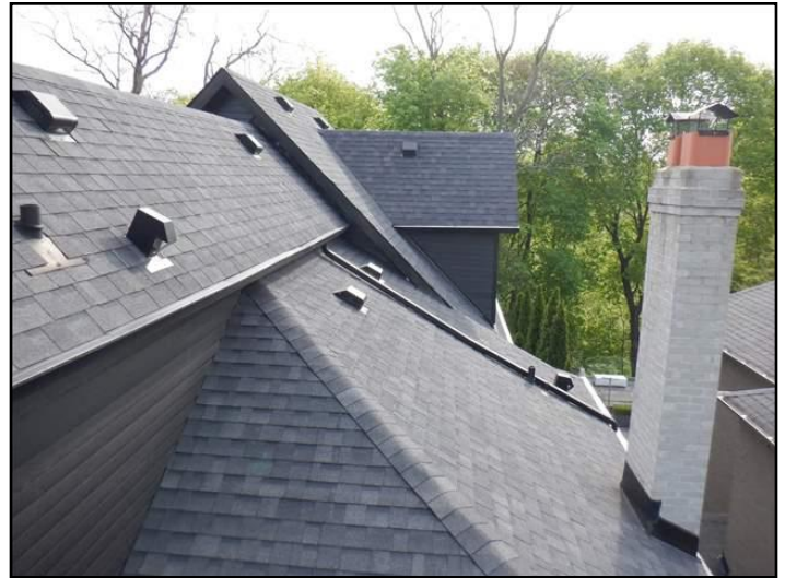
Asphalt shingles
