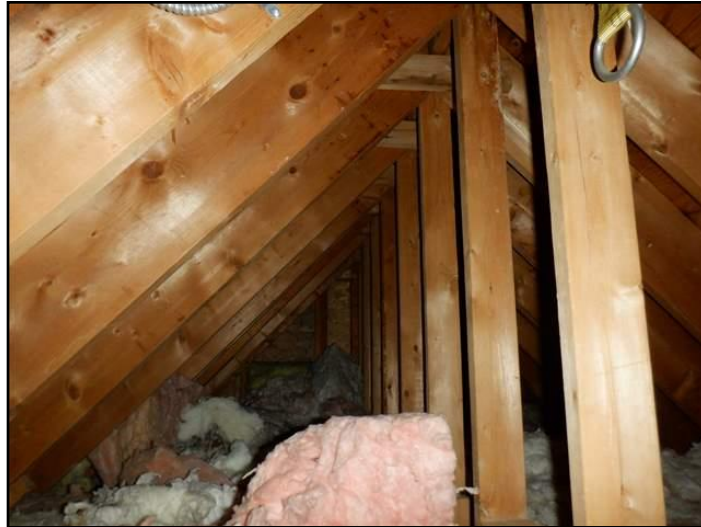
Rafters/roof joists
