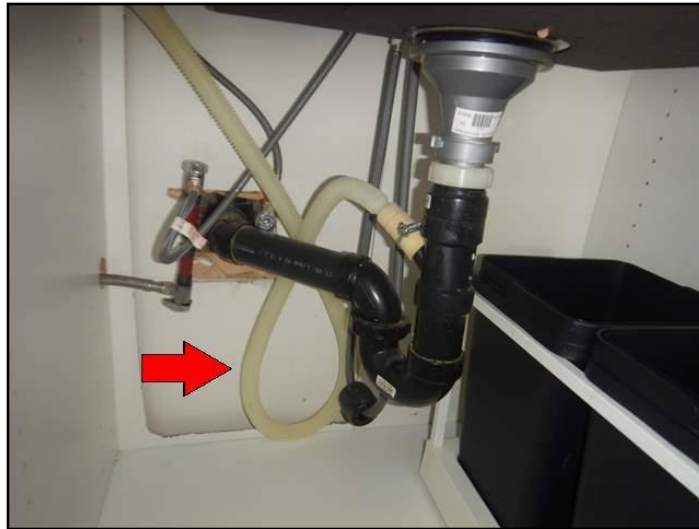
Dishwasher drain connections
