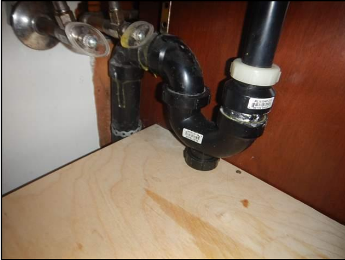
Example - First Floor Bathroom
